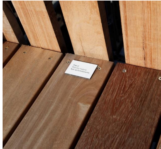
Pakoeli decking Kulbro View bridge Aarhus, 2017 Denmark (Source Mark van Benthem, Probos) https://www.lesserknowntimberspecies.com/cases/kulbro-view
